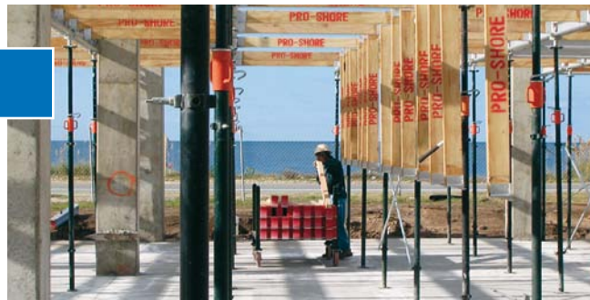
Joists are hung by one end from a ledger and then rotated into position at the opposite end by a single worker.
