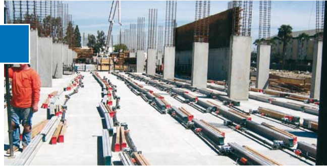
Staged components distributed from rolling carts in advance of erection.
