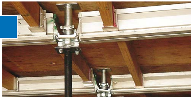
Dropheads shown released. Joists, ledgers, and plywood are freed so that 75% of the system can cycle to the next pour.
