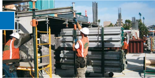
Ledgers are hung from the drophead on one end, then attached to the second post and raised into position by a single worker.
