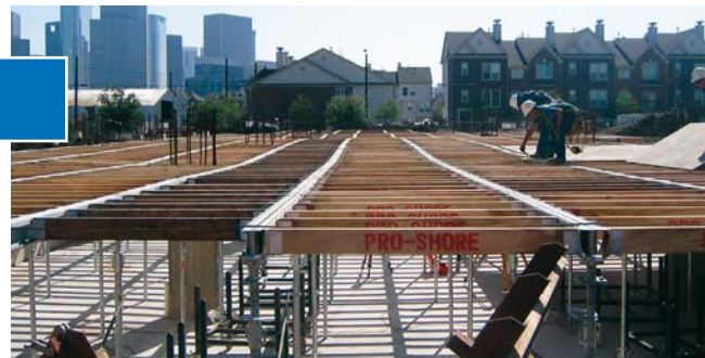
System is laser-graded using screw collars on the posts for fine adjustments, intermediate joists are added, and plywood panels are tacked in place with four 8-penny nails each.
