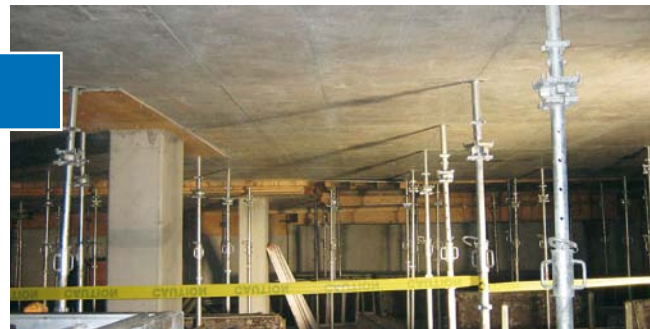
Posts reset in place serving as reshores after joists, ledgers, and plywood are stripped.
